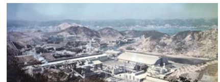
View of the completed copper refinery in 1969, including the new copper smelting plant
