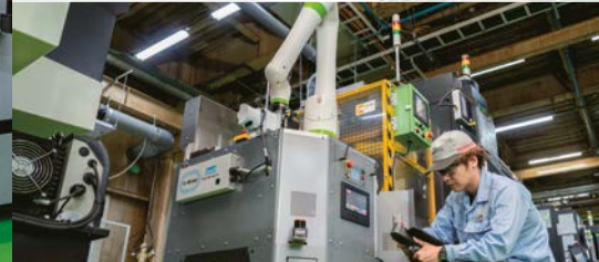
AMR (autonomous mobile robot) conducting an inspection.
