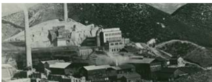
Naoshima Smelter & Refinery around 1932, immediately after starting operation
